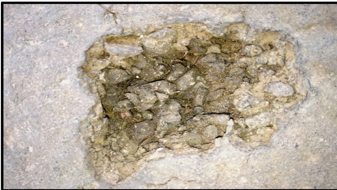
Fig.2 Typical Pot Hole in Pavement before Repairing.
