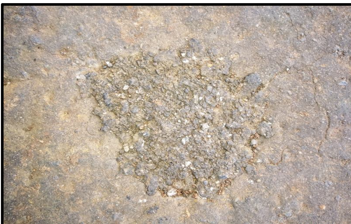
Fig.3 Pot Hole Repaired using WPA-Bitumen Mix.
