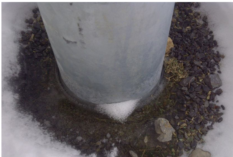
Figure 2. A pile moving out due to frost. The movement can be observed at the base of the pile.
