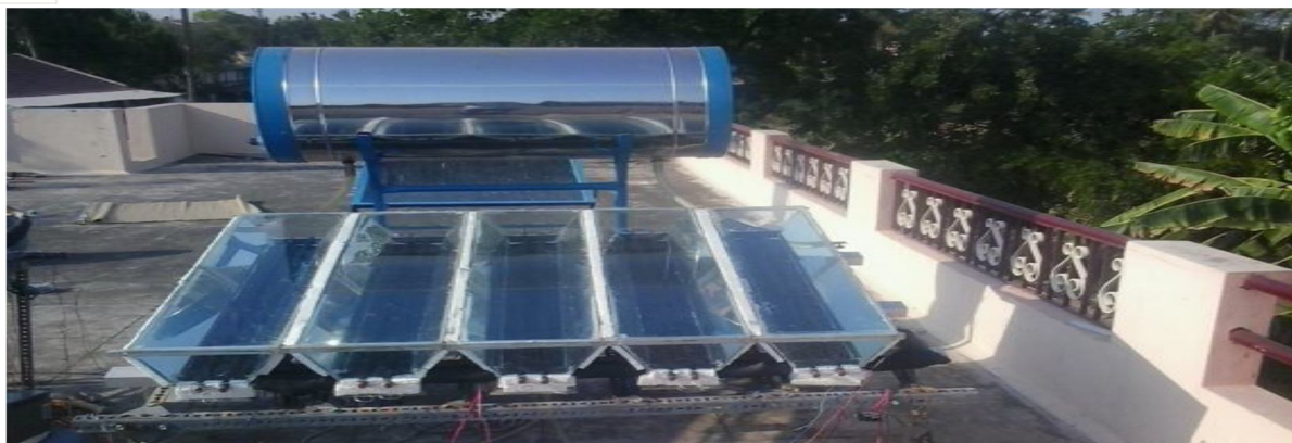
Fig no: 7 Construction of v-trough
