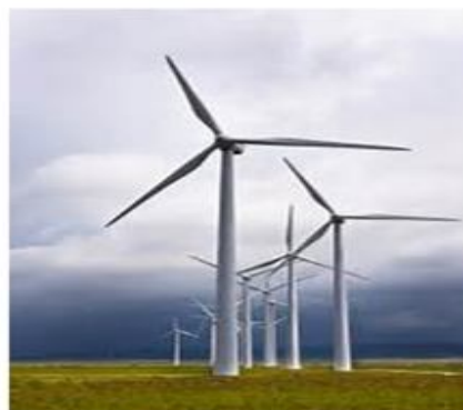
Fig 2: Traditional wind turbine
