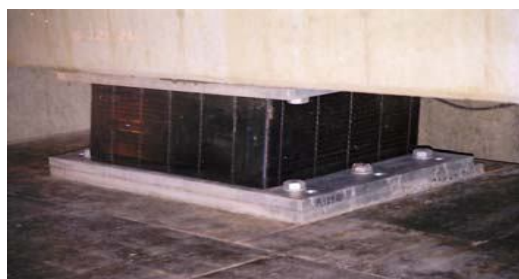
Fig. 6 High damping rubber bearing used in bridge
