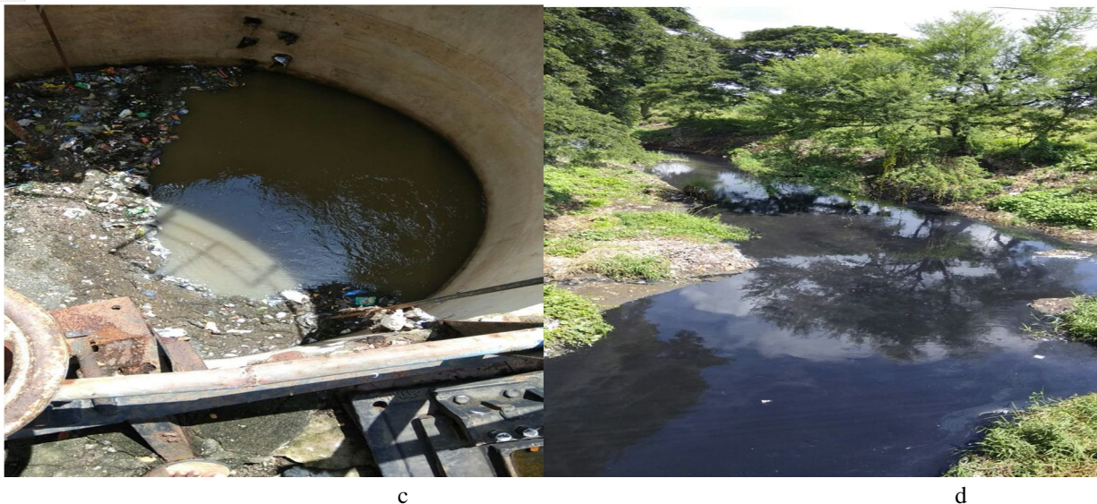
Fig.3. (a, b, c, d) Sewage treatment plant and Kala Nala
