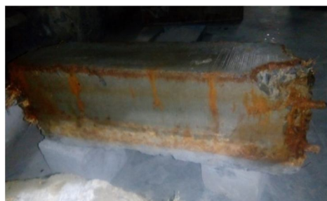
Fig.7 Corroded beam.
