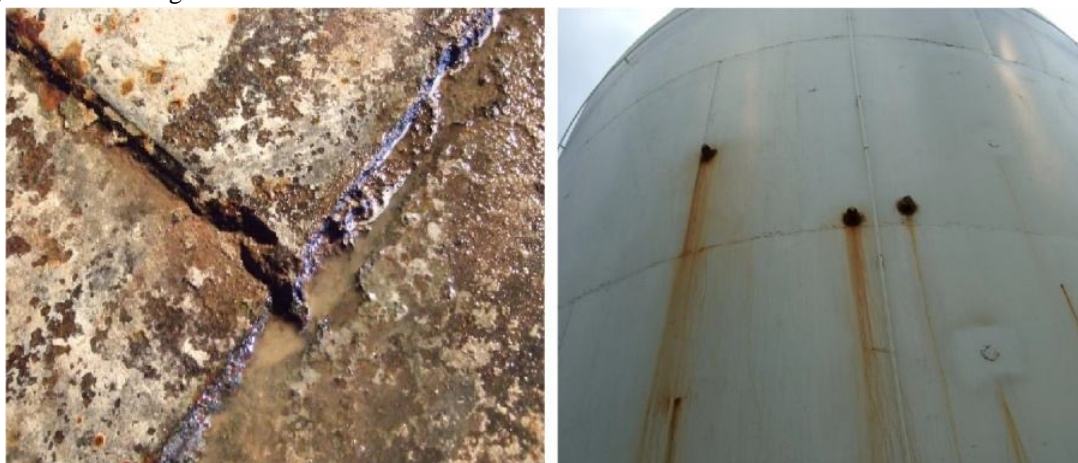
Fig. 1 Evidence of Shell Corrosion [13]
