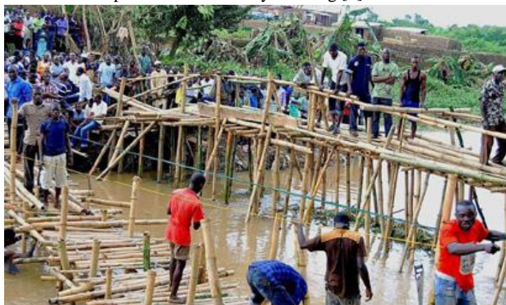
Fig. 2: showing Apete Pedestal Bridge under construction
