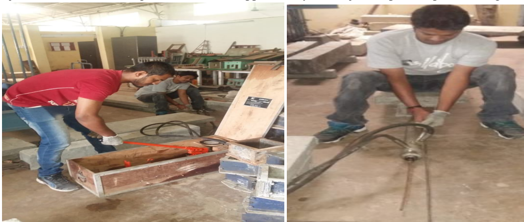
Figure.3. Post-tensioning of beams
