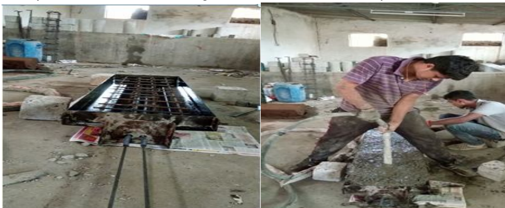
Fig 2:- Casting of Post Tensioned T- Beams
