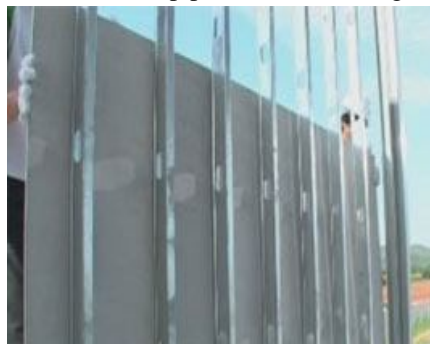
Fig. 4 Mounting 8mm SHERA board on one side
