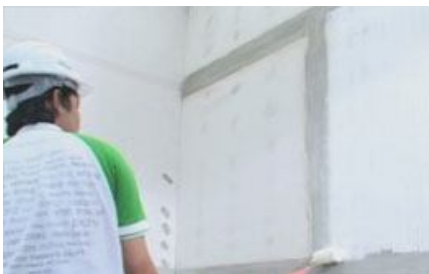
Fig. 8 Finishing of joints with Shera PU sealant.
