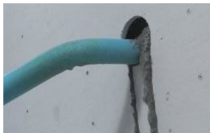
Fig. 7 Pumping light weight concrete from top
