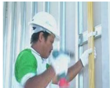
Fig. 4 Mounting 8mm SHERA board on one side
