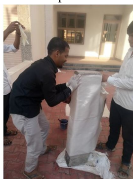
Application of GFRP sheets
