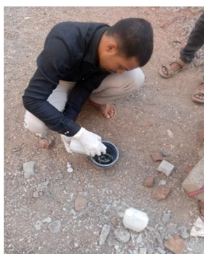
Mixing of epoxy primer
