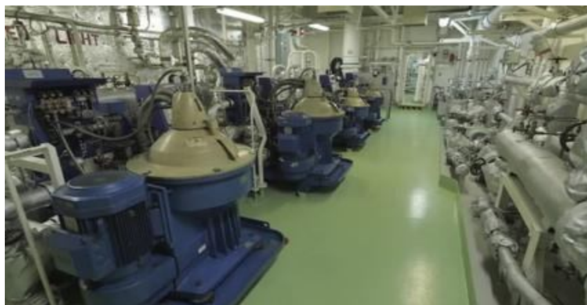
Fig 1: Centrifugal fuel oil separators[1]
