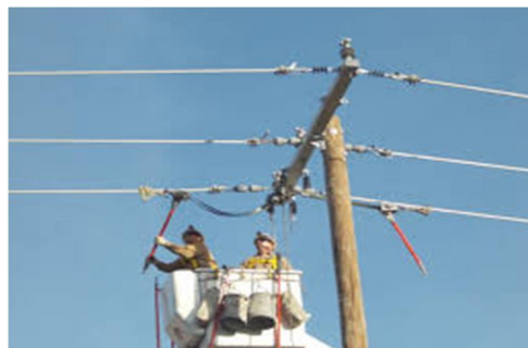
Fig.2 shows hot stick method using insulated sticks
