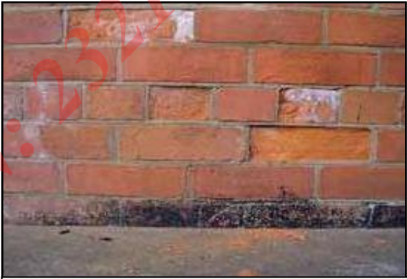
Photo No. 1. Affected Wall by Salinity
