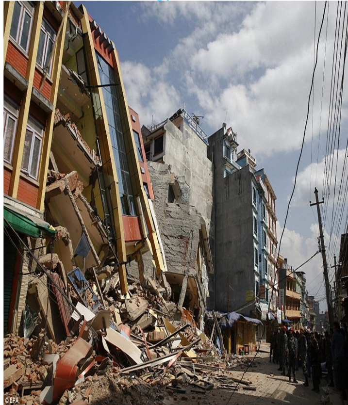
Figure 2: column, joints fail
