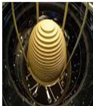
Fig: 4 Tuned mass Damper
