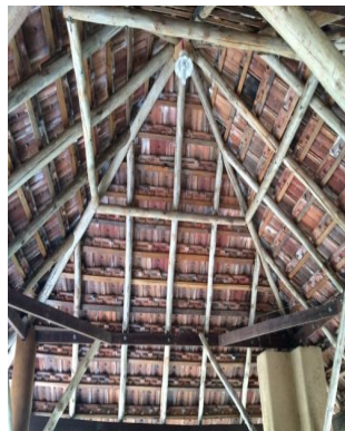
Fig. 6 Tiled roofing on Casuarina framed structure
