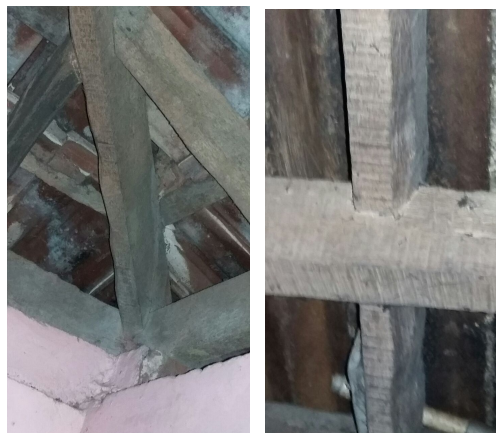
Fig. 8 Wall plate and rafter-purlin joinery
