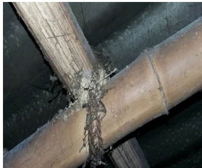
Fig. 10 Joinery using coir
