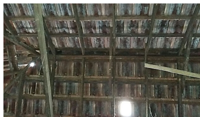
Fig. 7 Tiled roofing on coconut-framed structure
