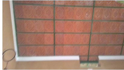
Fig. 3 Mangalore tiles laid exposed to the interior.
