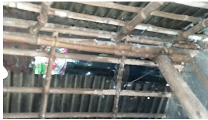
Fig. 9 Sheet roofing on bamboo-areca framed structure
