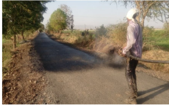
Fig-4 Bituminous mix lying on site
