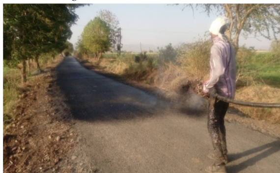
Fig-4 Bituminous mix lying on site
