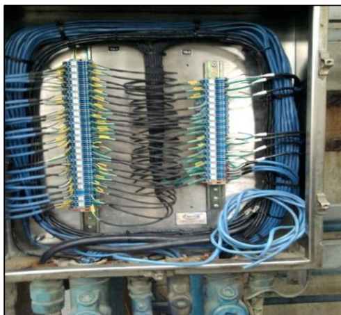
Fig. 7 Interior Junction Box Terminal.
