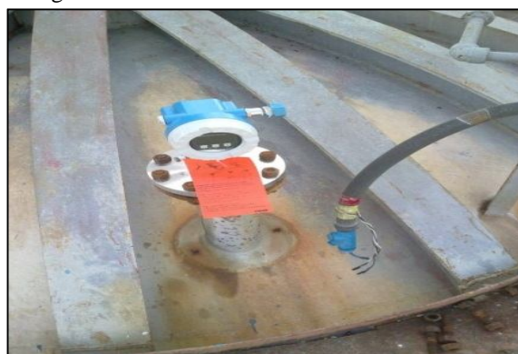
Fig. 5. New radar installed.
