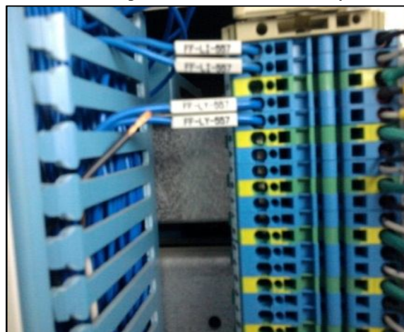
Fig. 11 Terminal block. Arrival of Radar Threads
