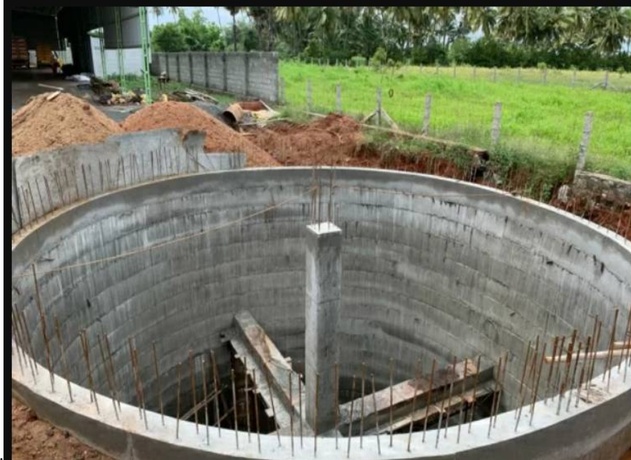
Fig. 1.3 RCC Circular Water Tank
