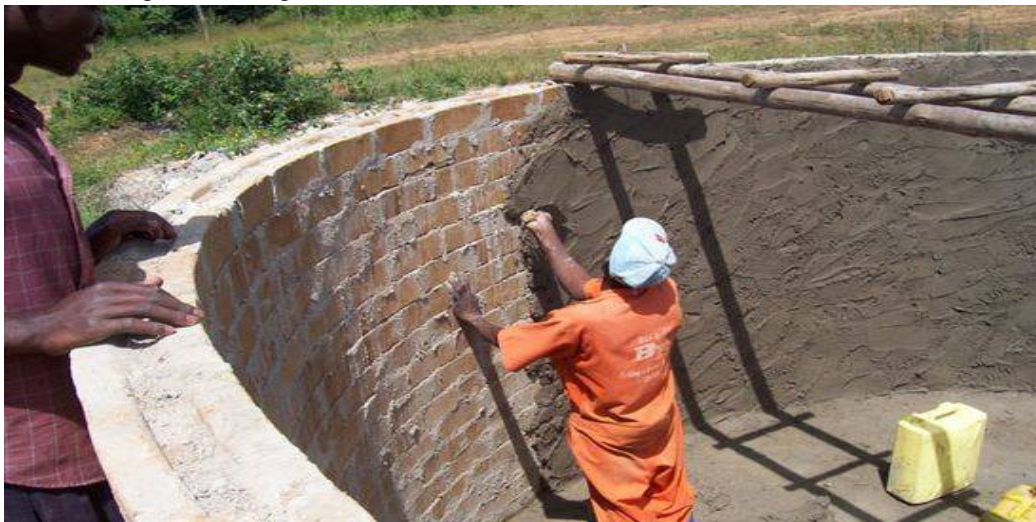
Fig. 1.1 Circular Water Tank
