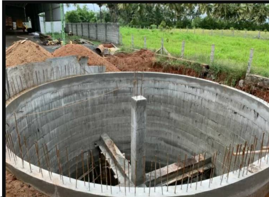
Fig. 1.3 RCC Circular Water Tank
