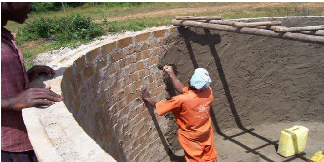
Fig. 1.1 Circular Water Tank
