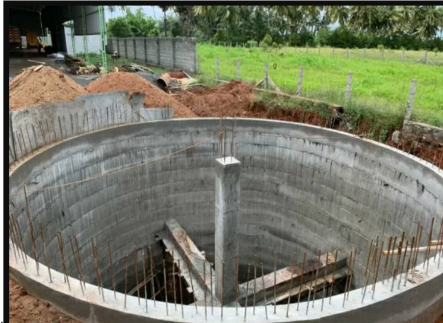
Fig. 1.3 RCC Circular Water Tank
