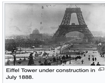
Fig. 3b. Eiffel Tower Under Construction
