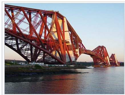
Fig. 3a. The Forth Bridge
