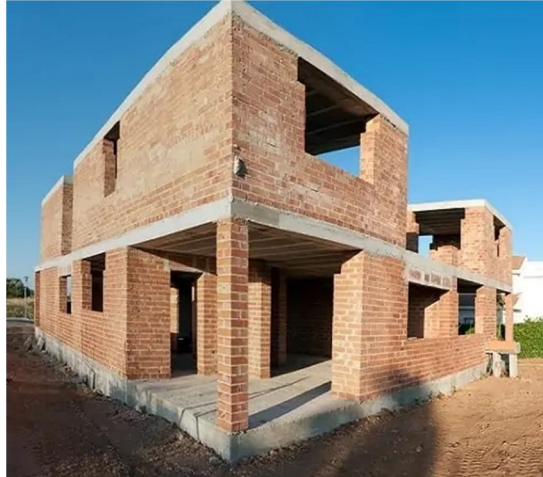
Fig. 6. Load Bearing Structure
