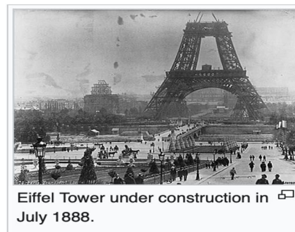
Fig. 3b. Eiffel Tower Under Construction
