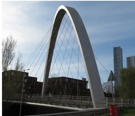
Fig. 10. Cables and Arche Structure
