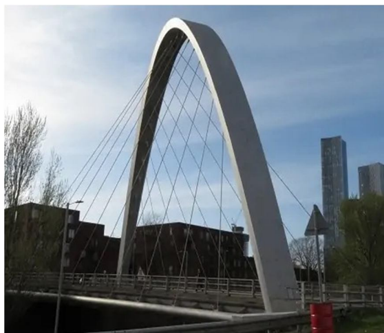
Fig. 10. Cables and Arche Structure
