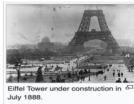
Fig. 3b. Eiffel Tower Under Construction
