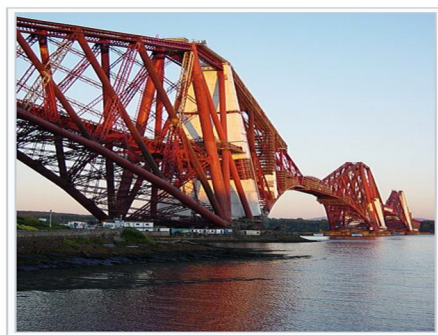
Fig. 3a. The Forth Bridge
