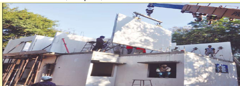
Figure 2 Construction of GFRG panel house
