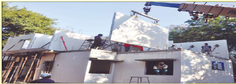
Figure 2 Construction of GFRG panel house
