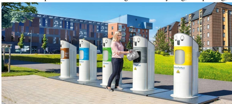
Fig 11. Pneumatic waste collection
