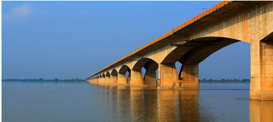
Fig -1: Ganga Sethu Bridge Patna
