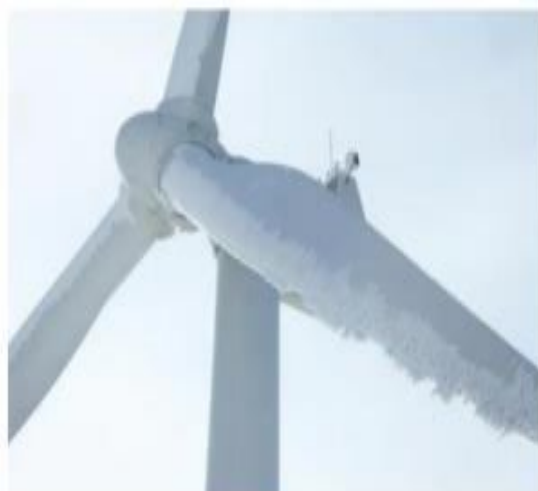
Figure7: Icing on the wind turbine.
