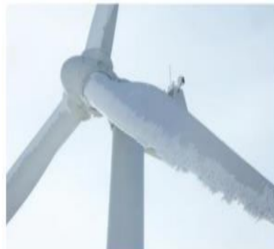
Figure7: Icing on the wind turbine.
