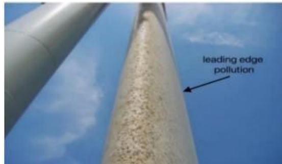
Figure 6(a): Pollution on wind turbine.
