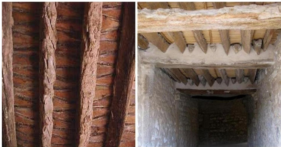
Fig. 7 Use of palm (trunk and leaves) in construction [68]
