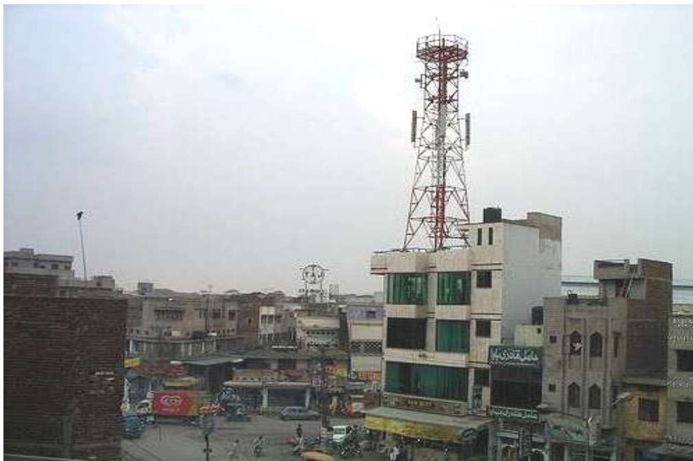
Fig. 1: Structure with Telecommunication tower at top
