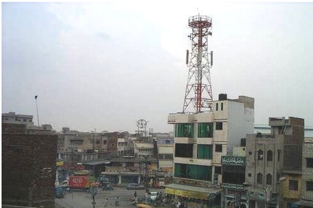
Fig. 1: Structure with Telecommunication tower at top
