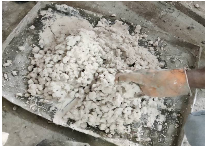
Figure 4.5: Mixing of MOC concrete
