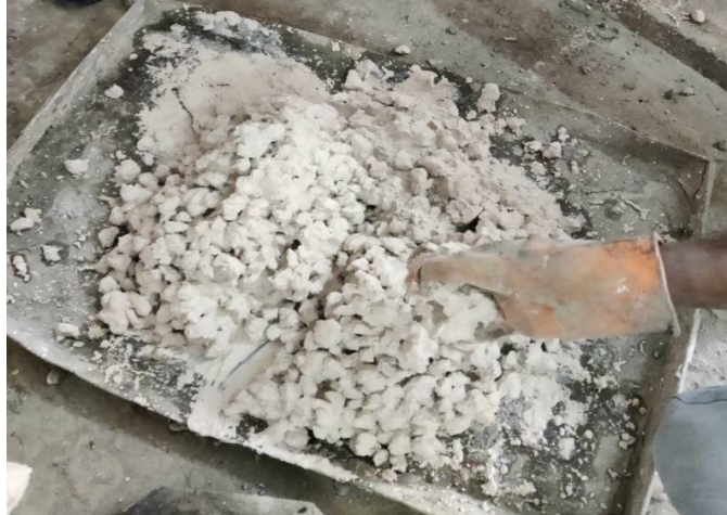
Figure 4.5: Mixing of MOC concrete
