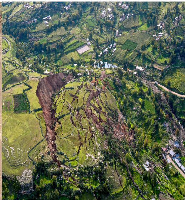
Fig. 6b. Sliding Planes near Cusco, Peru in 2018 Top Right) used to Form a Single Continuous Line, but have been Split Apart by Movement along the Fault
