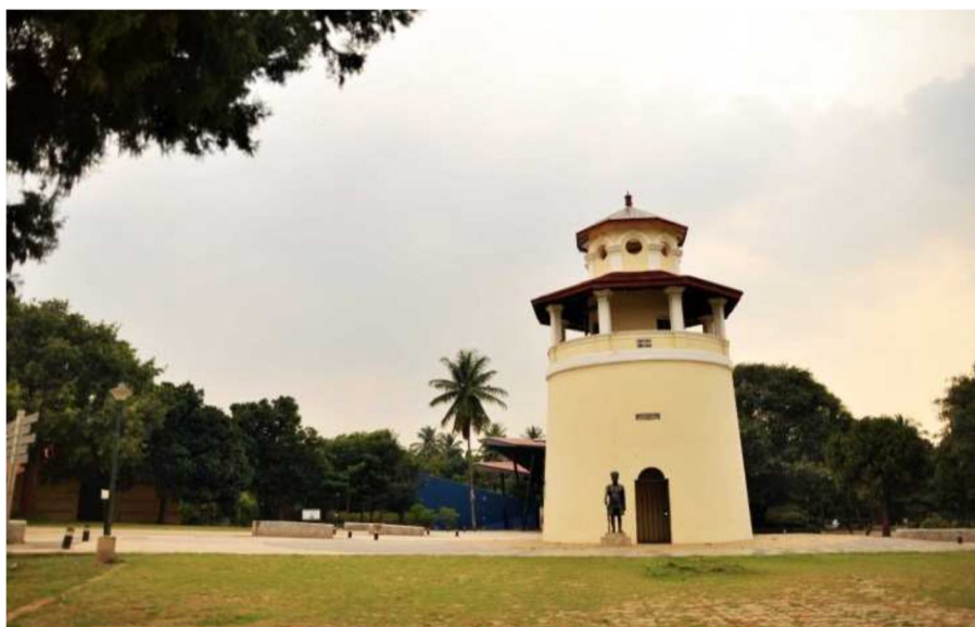
Fig 4: The reused “watchtower”
