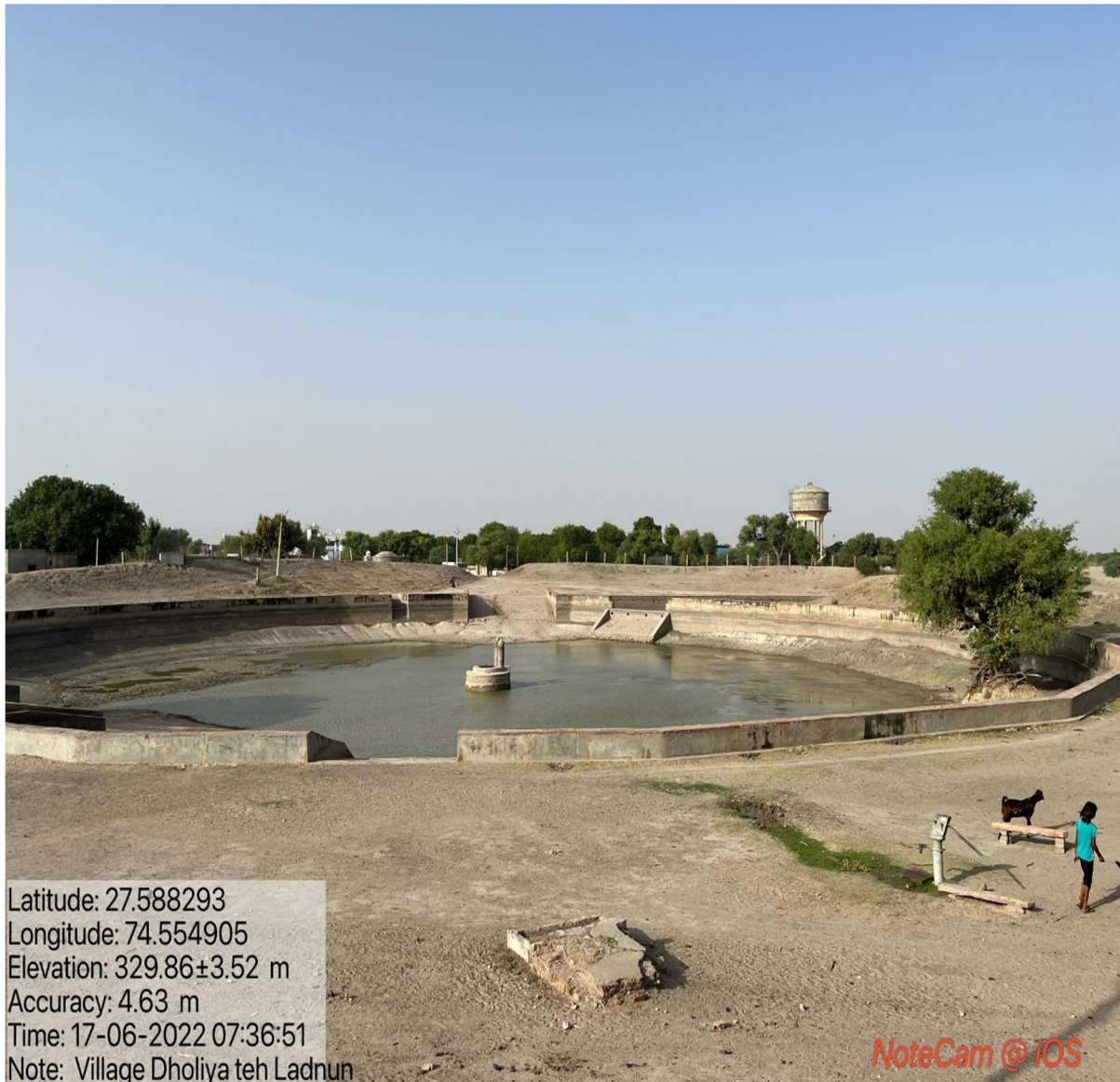
Figure: 6. Viable water harvesting structure in Ladnun block, Nagaur District of Rajasthan
