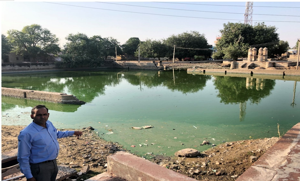
Figure: 7. Viable water harvesting structure alongside an Open Well in Ladnun block, Nagaur District of Rajasthan
