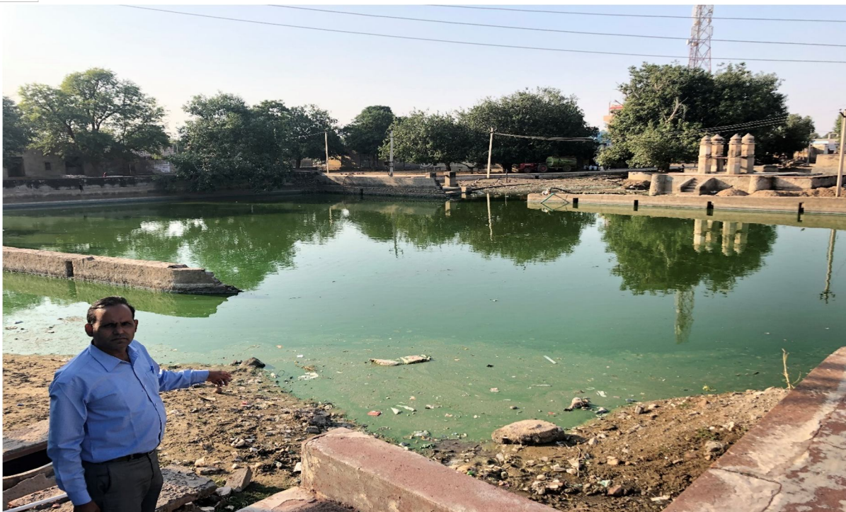
Figure: 7. Viable water harvesting structure alongside an Open Well in Ladnun block, Nagaur District of Rajasthan
