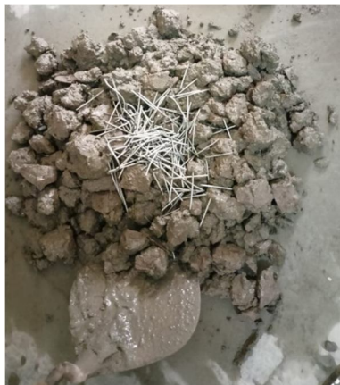
Fig:3 Mixing Of GI Wire
