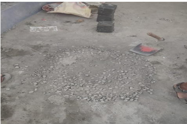
Fig 1: Dry mixing
