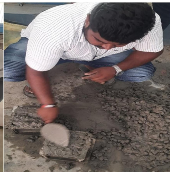
Fig 4: pouring of concrete
