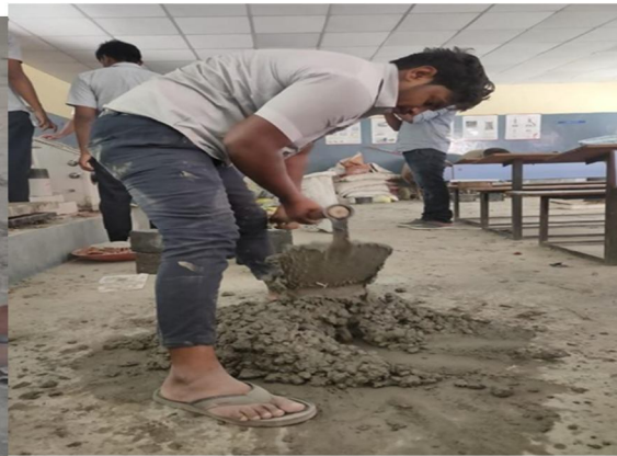
Fig 2: Wet Mixing
