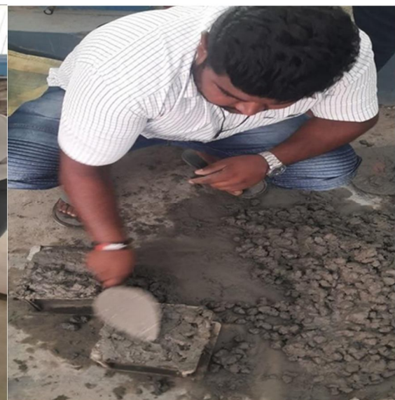
Fig 4: pouring of concrete
