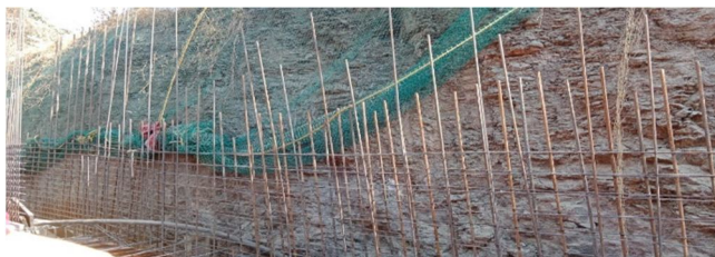
Figure:3 site at wagholi, Pune
