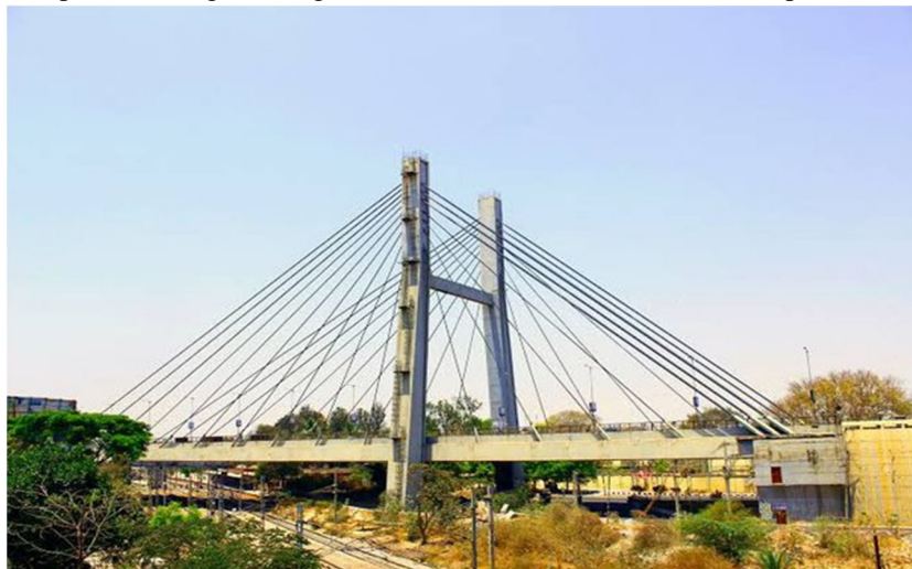
Fig 2: Cable stayed bridge
