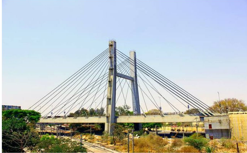
Fig 2: Cable stayed bridge
