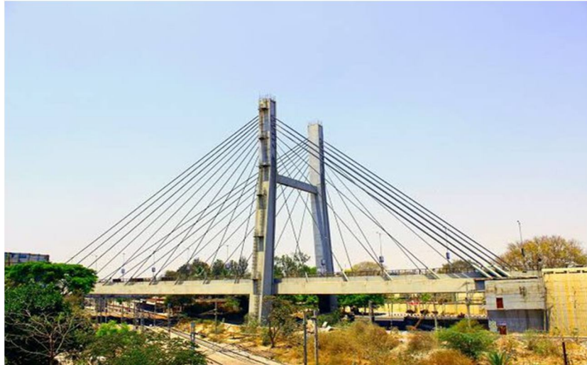
Fig 2: Cable stayed bridge
