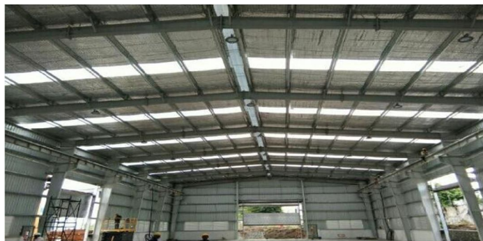
Fig. 1: Pre-Engineered Warehouse Structure
