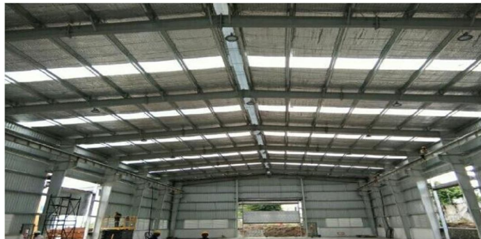
Fig. 1: Pre-Engineered Warehouse Structure
