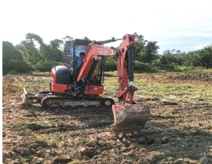
Figure 10: Use of Kubota mini farm excavator
