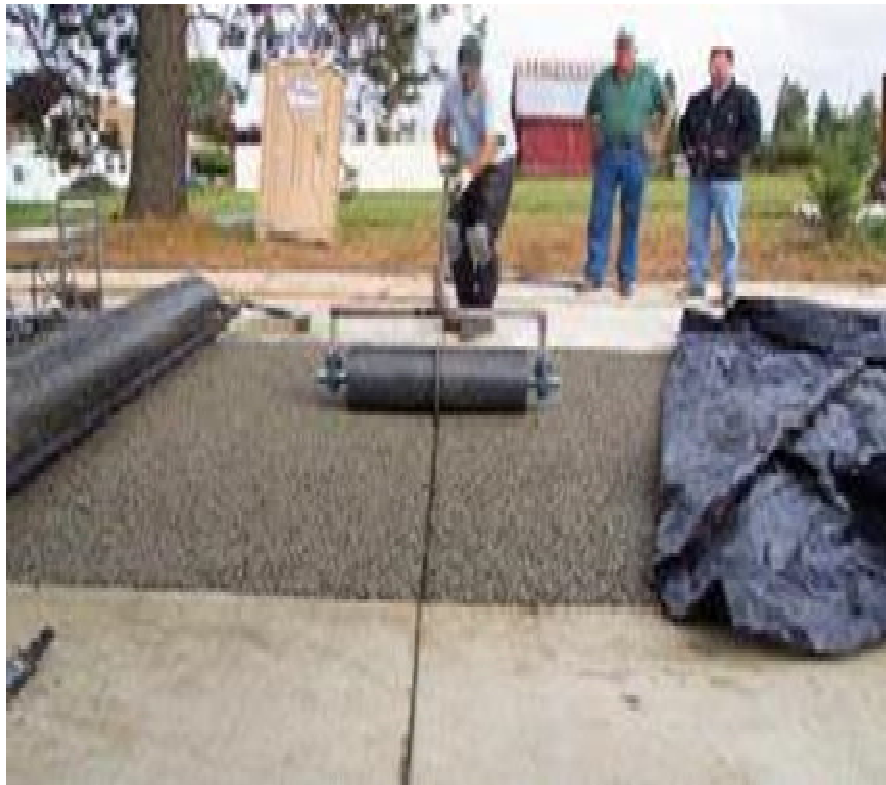
Fig7 Joint rollers, commonly referred to as a “pizza cutter.”
