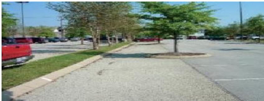
Fig.2 pervious concrete pavements for parking lots
