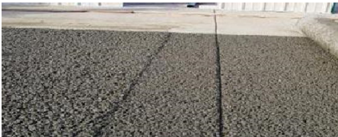
Fig 5 Pervious concrete after screeding (left) and after compaction (right)
