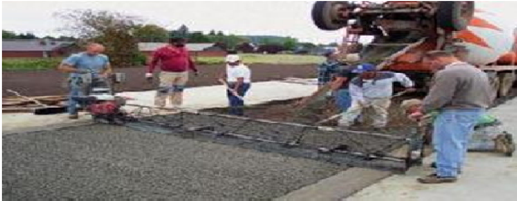
Fig 4 Pervious concrete is usually placed and then struck off
