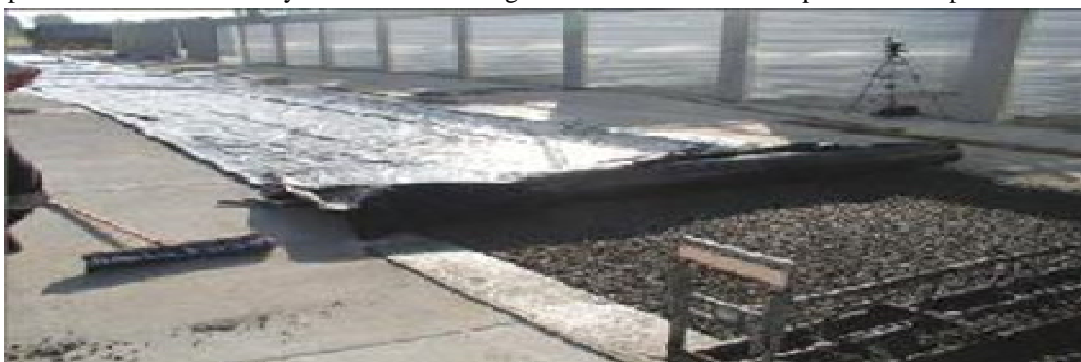
Fig 8 Plastic sheeting should be used to cover the pervious concrete and be installed within a few minutes of consolidation to Prevent moisture loss
