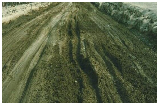
Figure 8 Formation of ruts in un reinforced section
