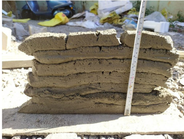
Figure 4: Checking the shape of printed concrete for deformations if any
