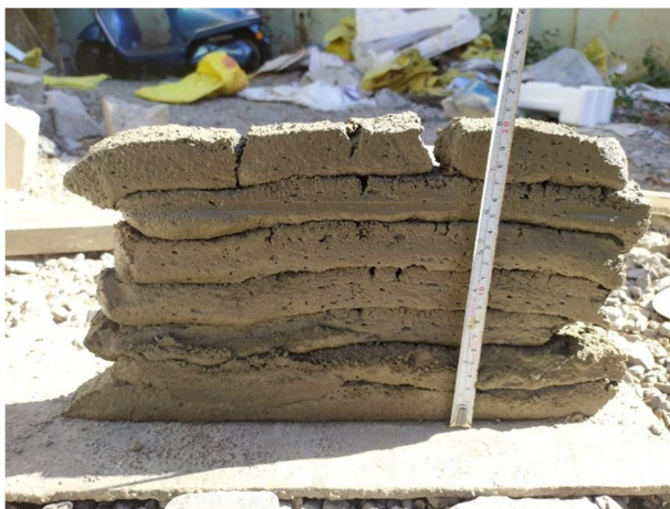
Figure 4: Checking the shape of printed concrete for deformations if any
