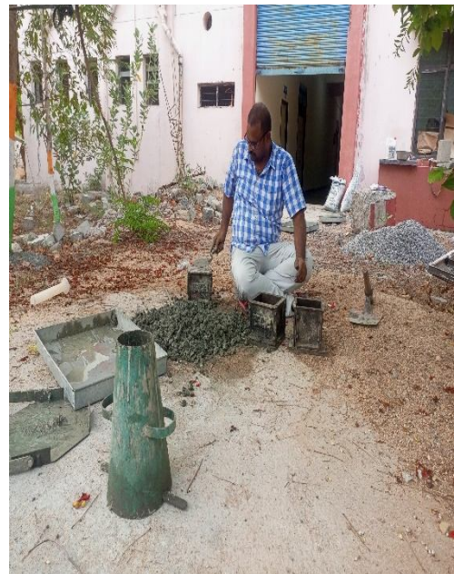
Fig. 4 Concrete Cube casting
