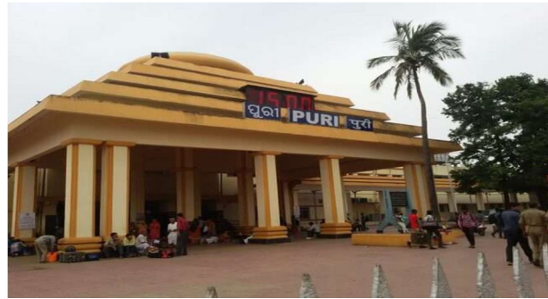
Image 2: Puri Railway Station, Puri, Odisha
