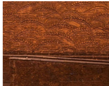
Fig.49: Terracotta Inlay in Walls
