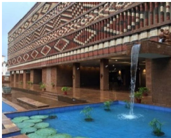
Fig.48: Exposed Brick Structure
