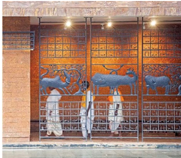
Fig.45: Wrought Iron Partitions
