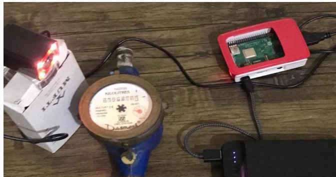
Fig. 5 Automated Water Meter Reading System
