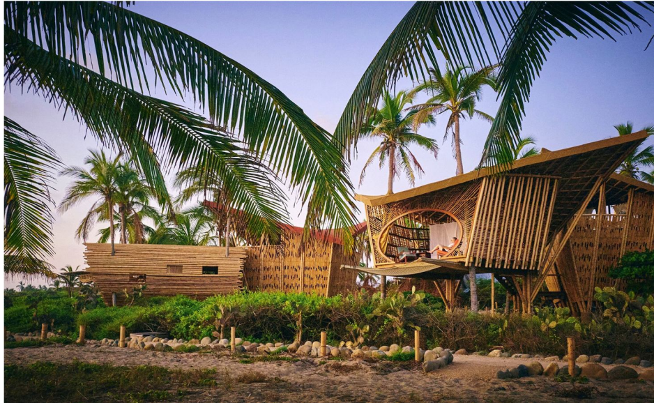
Fig 1: Use of bamboo poles and folded bamboo strips in a bamboo house
