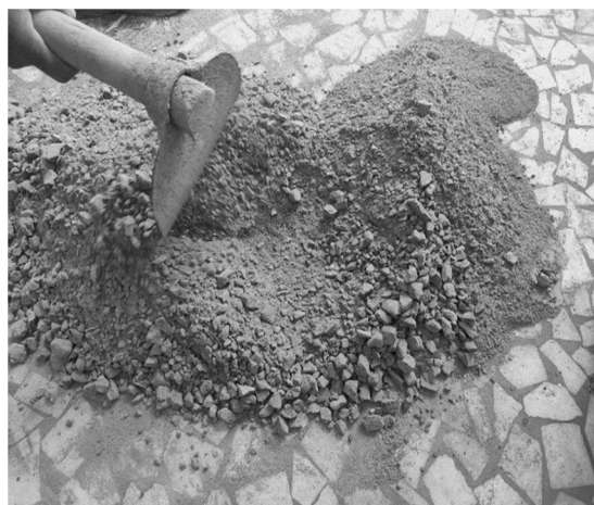
Fig.5.2.1.1 Mixing of materials
