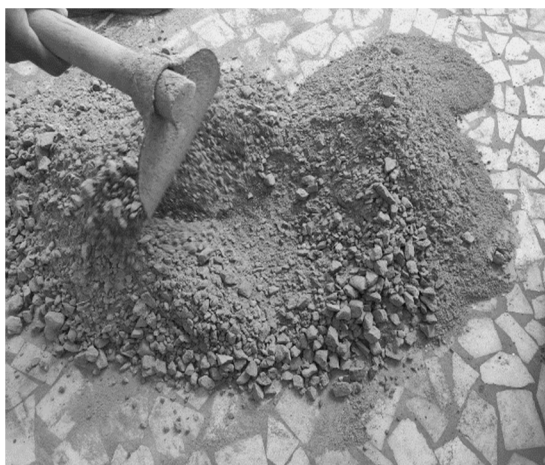
Fig.5.2.1.1 Mixing of materials
