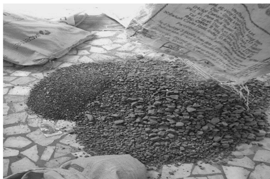
Fig.5.2.1 Mixing of materials
