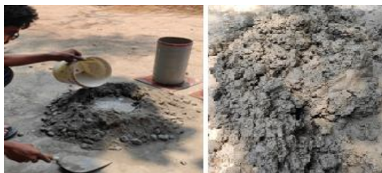
Fig. 6 Mix of concrete
