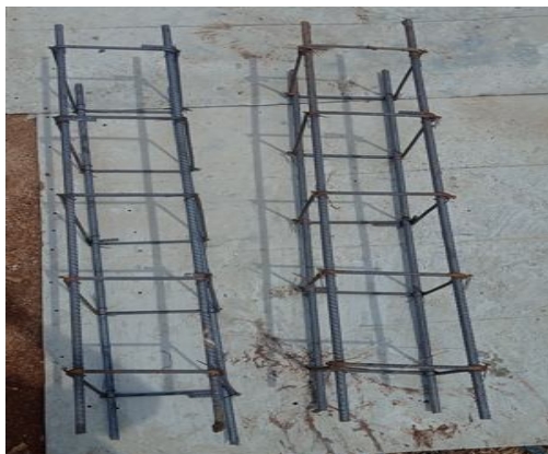
Fig. 8 Reinforcement Work of Column
