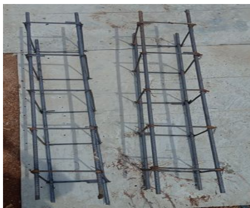
Fig. 8 Reinforcement Work of Column
