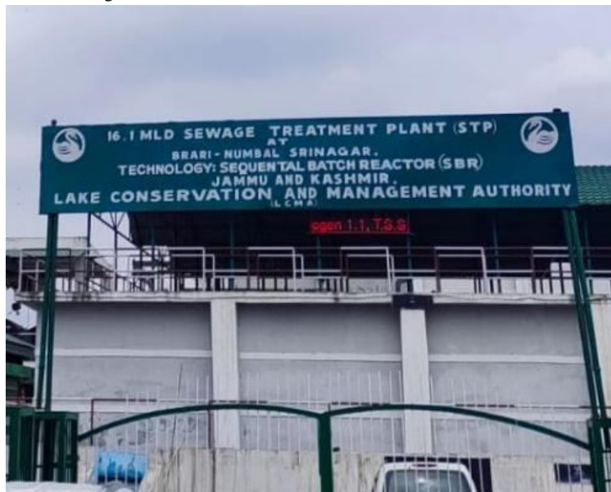
Figure 1: Sewage Treatment Plant Brari Nambal
