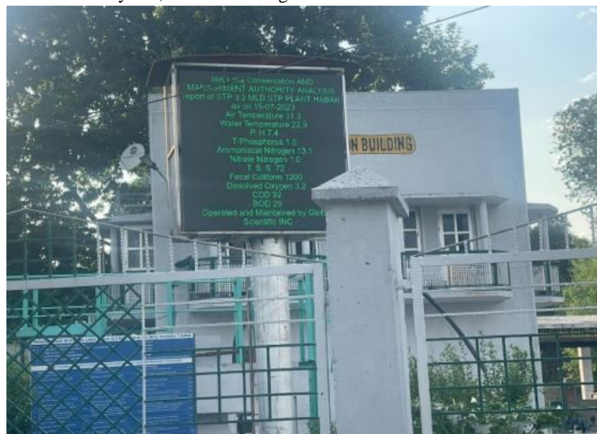
Figure 2: Sewage Treatment Plant Habak
