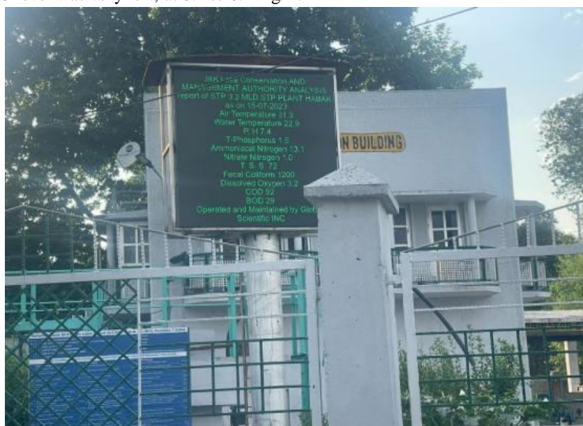
Figure 2: Sewage Treatment Plant Habak
