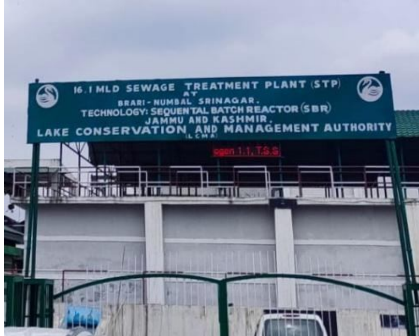
Figure 1: Sewage Treatment Plant Brari Nambal
