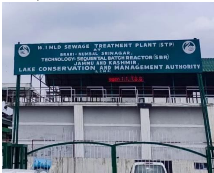
Figure 1: Sewage Treatment Plant Brari Nambal
