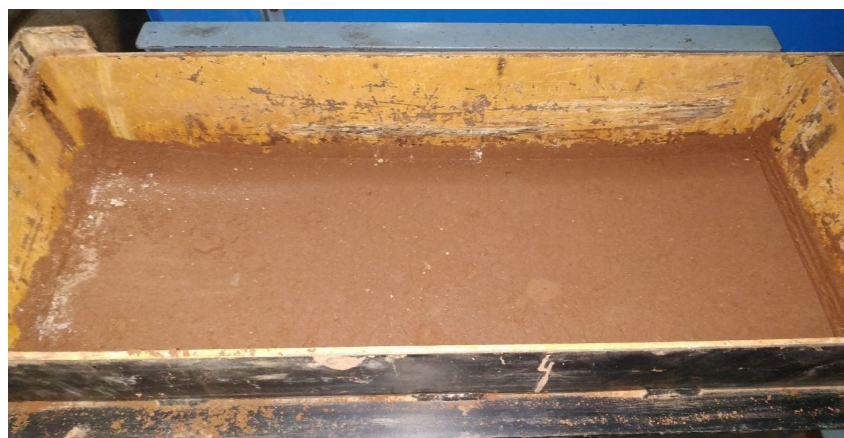
Fig. 2 Compacted Sub Grade
